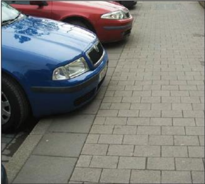
01- An example where a narrow verge is provided to ensure that vehicle overhangs do not intrude on the footway (Figure 4.36 DMURS)
